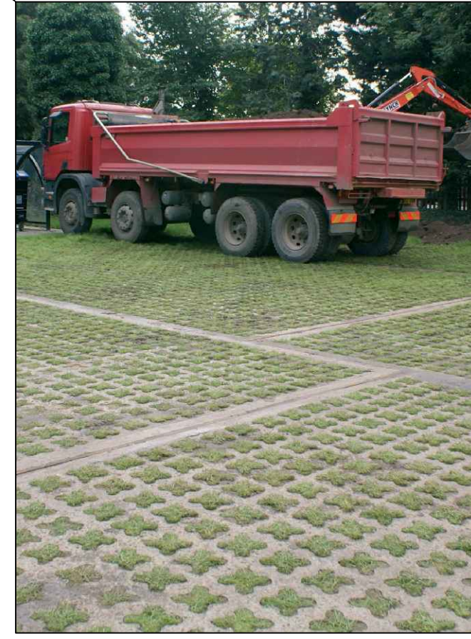
TYPICAL GRASSCRETE PAVING AFTER INSTALLATION
